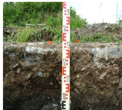
Figure A.5 Levelling Staff in Close-Up
