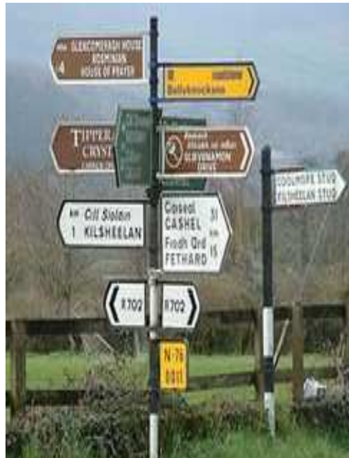
Too many signs on one post can be confusing and unclear.
