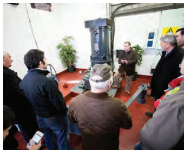
Photo 7: Officials and Elected Members inspect a Hydro turbine on the River Suir at Holycross (Source-TEA)
