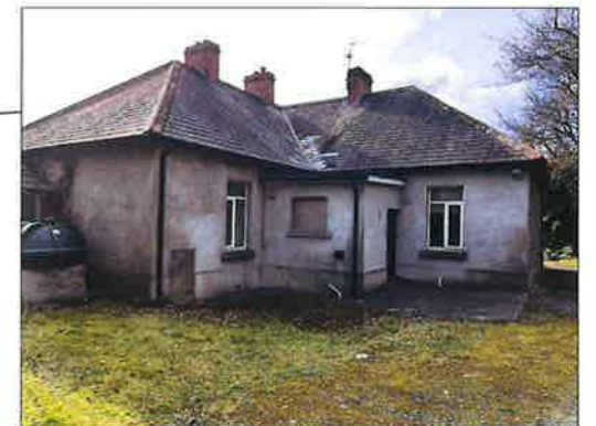
EXISTING UN-INSULATED FLAT ROOF BLOCK-WORK EXTENSION
