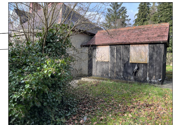
UN-INSULATED LIGHTWEIGHT TIMBER EXTENSION
