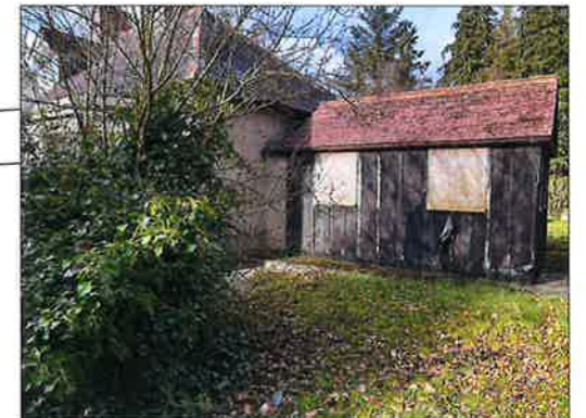
UN-INSULATED LIGHTWEIGHT TIMBER EXTENSION
