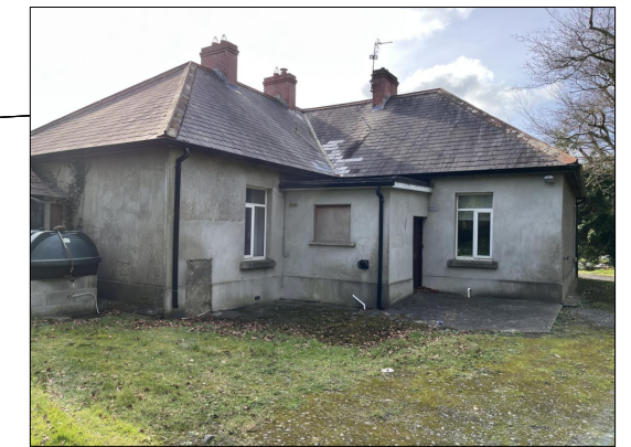
EXISTING UN-INSULATED FLAT ROOF BLOCK-WORK EXTENSION
