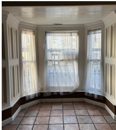
Examples of timber casing and window shutters within existing kitchen area at ground floor
