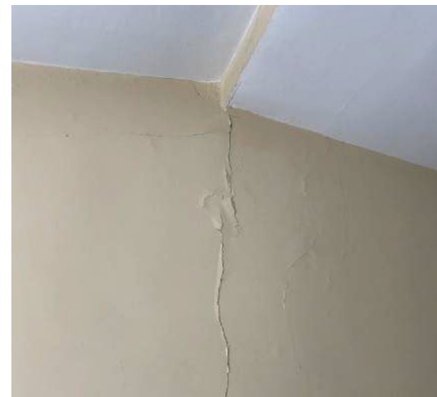
Cracking to internal and external wall finishes which could suggest historic movement.
