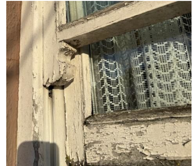
Example of condition of 1990s timber sash windows.
