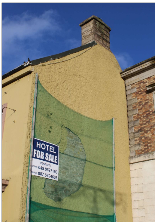
Plate 1: East gable end with collapsed area of render exposing rubble masonry stone construction
