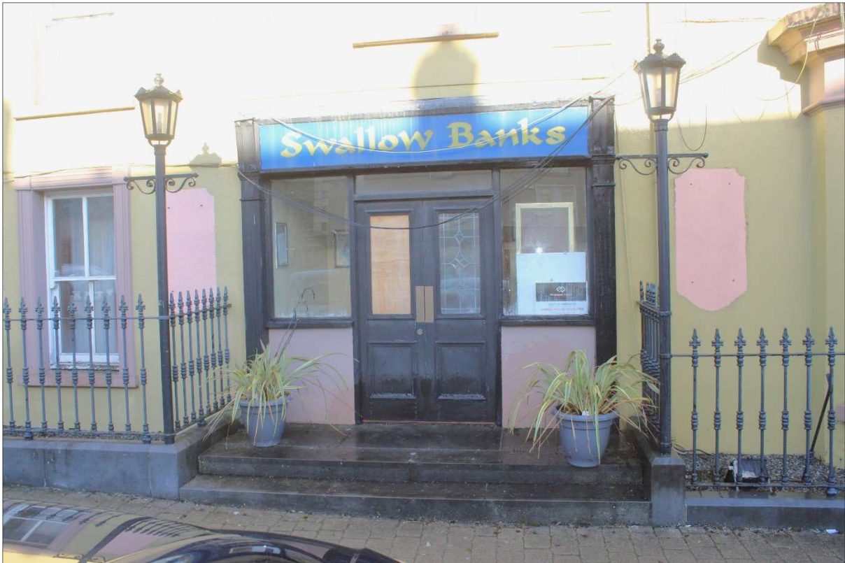
Plate 7: Infill doorway within former three-centred arch-headed opening to laneway formerly leading to stables and outbuildings to rear of site
