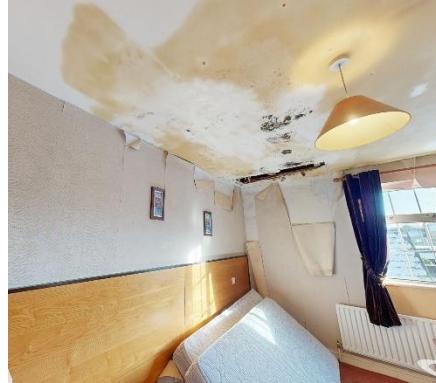
Decorative disrepair caused by water ingress
