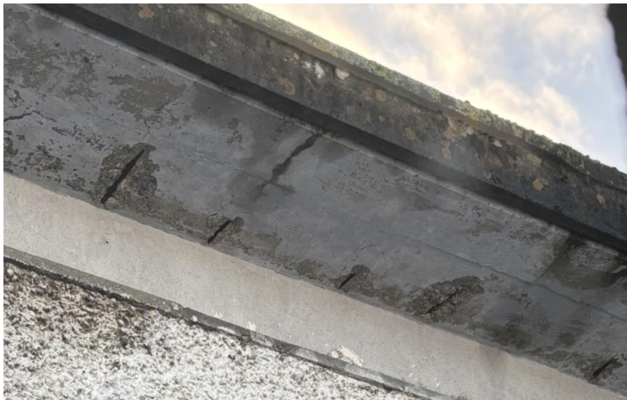
Rebar exposed to in situ concrete soffits at second floor
