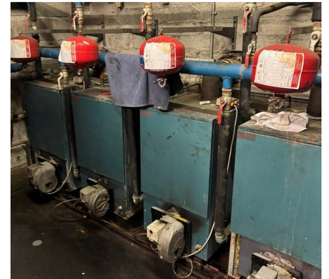
4no existing oil boilers have reached the end of their serviceable life and have high carbon emissions.
