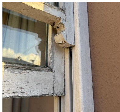
Examples of condition of 1990s windows. Top left – historically detailed single glazed window unit to existing kitchen area
