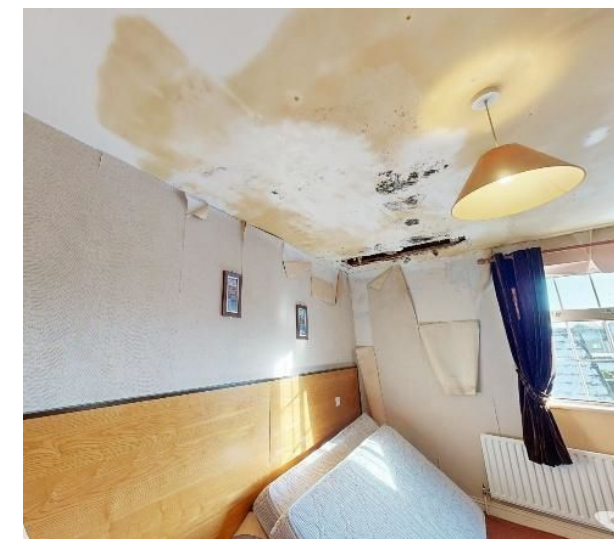
Decorative disrepair caused by water ingress.
