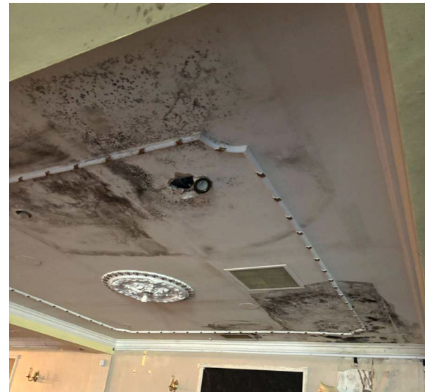
Water ingress to main function room at ground floor from failure of existing flat roof above.
