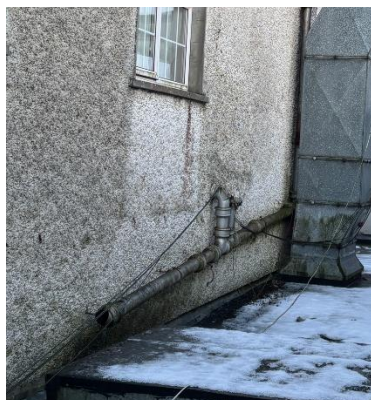
Damage to existing soil pipes
