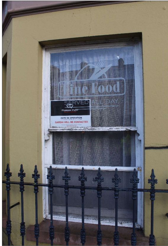
Plate 3: Detail of historic timber window frame with additional secondary glazing fitted over the lower sash
