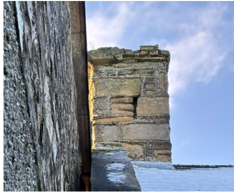
Damage to existing chimney
