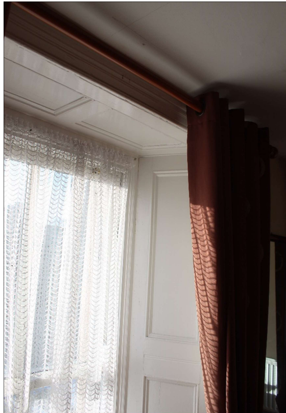
Plate 21: Detail of historic, timber panelled shutters and surround to interior of replacement window frames
