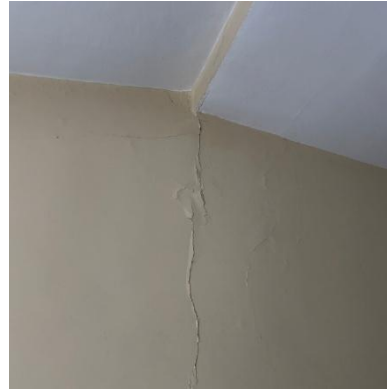
Cracking to internal and external wall finishes
