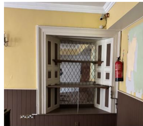
Existing bay window blocked up into former archway
