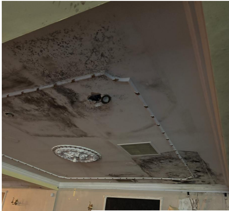
Water ingress to main function room at ground floor
