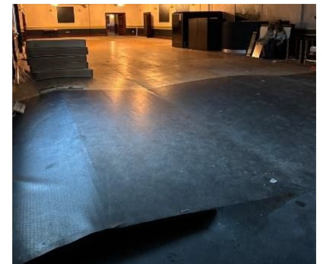
Significant buckling of function room floor.
