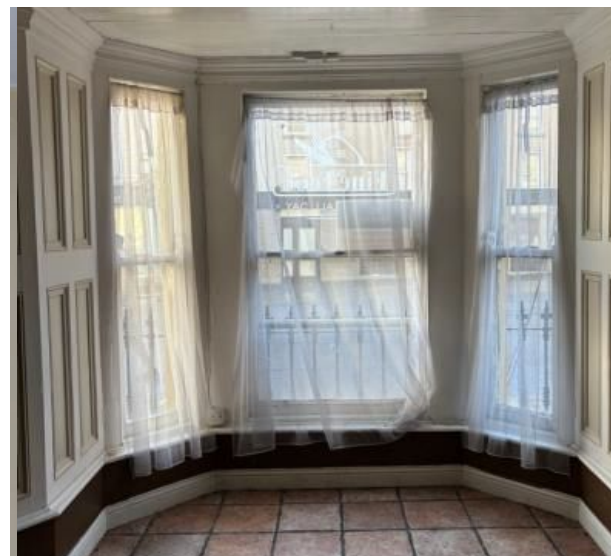
Examples of timber casing and window shutters within existing kitchen area at ground floor are some of last remaining original construction
