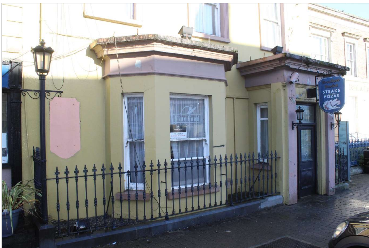
Plate 2: Wrought and cast-iron railings on limestone plinth to front elevation of building to east side of Castle Street façade. One-over-one timber sliding sash windows on canted bay here are among oldest surviving on site.
