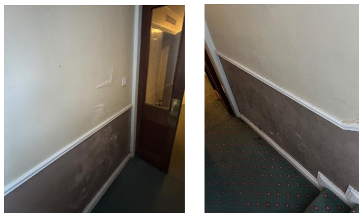
Blistering and peeling to finishes, and penetrating damp to first floor bedroom corridor
