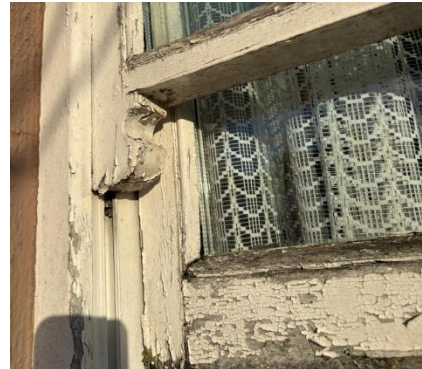
Examples of condition of 1990s windows. Top left – historically detailed single glazed window unit to existing kitchen area
