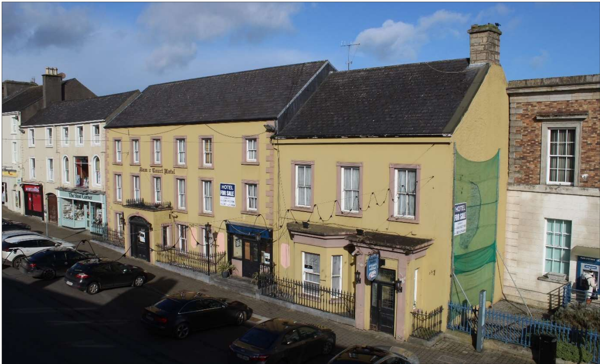
Figure 1: Cream-mustard coloured nine-bay south façade and east gable elevations of existing former hotel buildings to subject site on Castle Street. Note loss of all but one chimney stack to the eastern gable wall, replacement of all but three timber sash windows on the ground-level canted bay and apparent raising of all eaves lines across the Castle Street façade since the 1955 aerial photograph of the site shown below in figure 4 .
