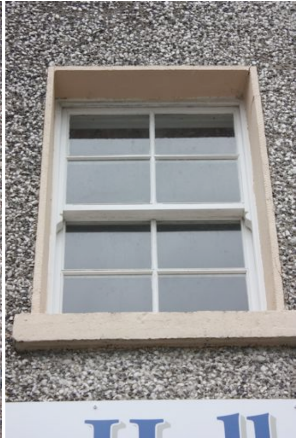
5. North room ground floor window, six over six sliding sash window, patent reveals and cut stone cill with severe cracking. 6. First floor north room window, four over four sliding sash window.
