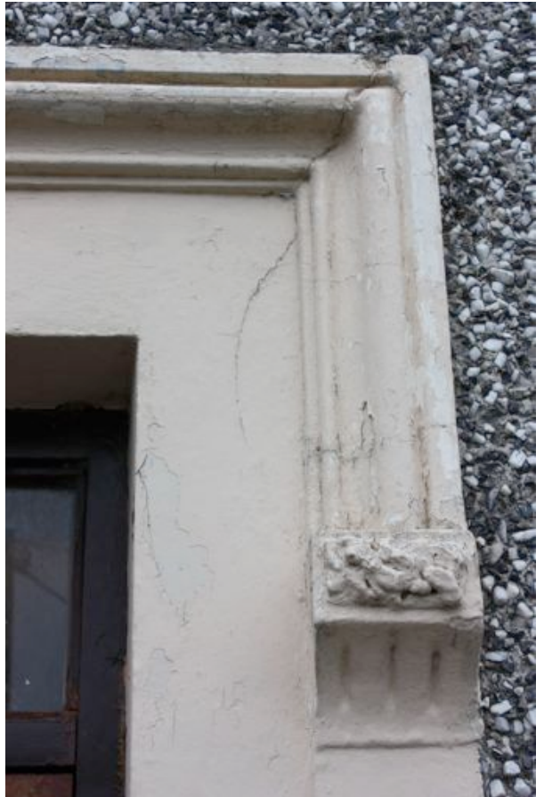
3. Front door and surround, modern replacement six panel hardwood door, original frame and fanlight retained. Sand-cement surround with hood moulding and brackets. 4. Detail of hood moulding and bracket to entrance door.
