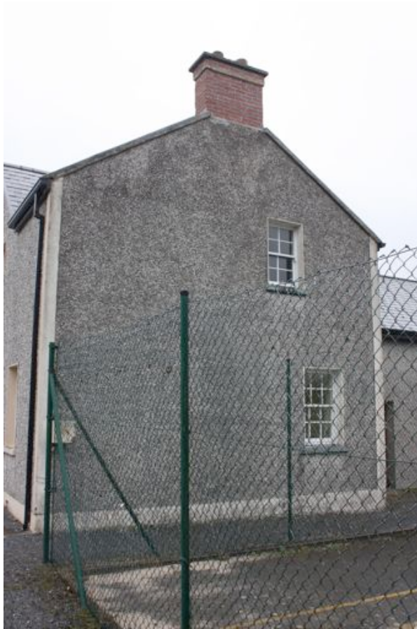
9. South gable of house. 10. South-east corner of house, plain render reveals with pebble-dashed finish, replacement rainwater goods and fascias.
