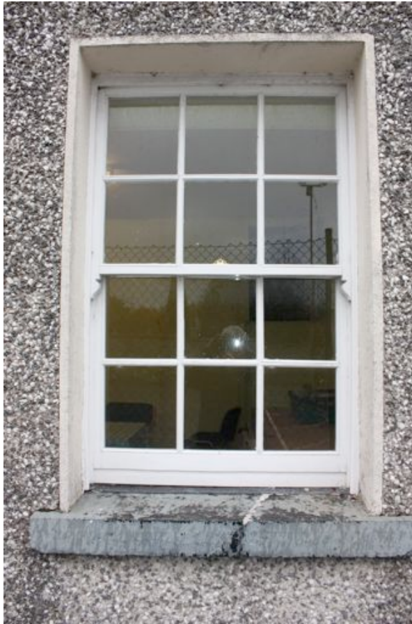
5. North room ground floor window, six over six sliding sash window, patent reveals and cut stone cill with severe cracking. 6. First floor north room window, four over four sliding sash window.
