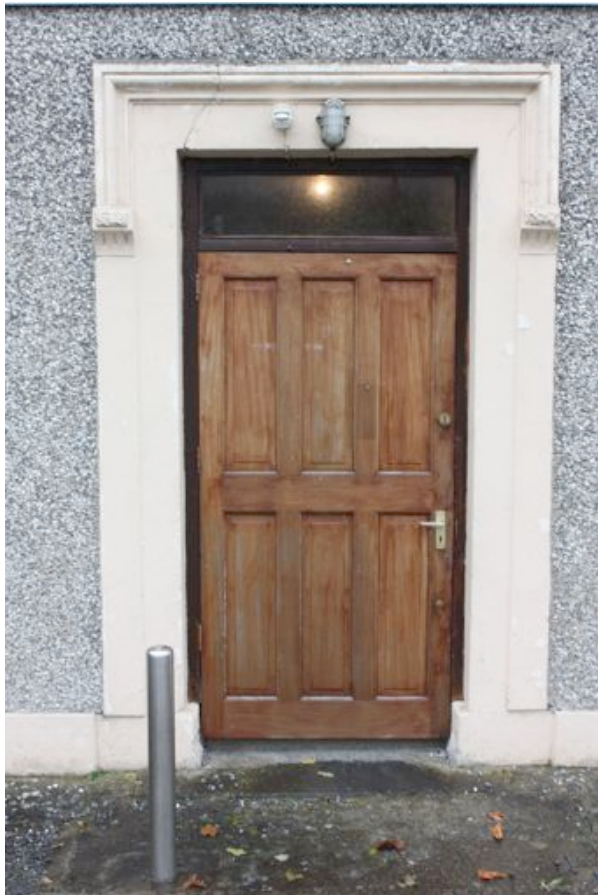
3. Front door and surround, modern replacement six panel hardwood door, original frame and fanlight retained. Sand-cement surround with hood moulding and brackets. 4. Detail of hood moulding and bracket to entrance door.
