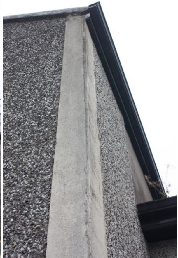
9. South gable of house. 10. South-east corner of house, plain render reveals with pebble-dashed finish, replacement rainwater goods and fascias.
