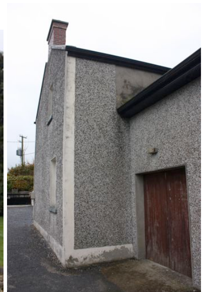
11. East gable of community hall with house in background. 12. East (rear) wall of original house with community hall abutting the original wall. Note, the portion of the original wall directly above the community hall roof is not pebble-dashed.
