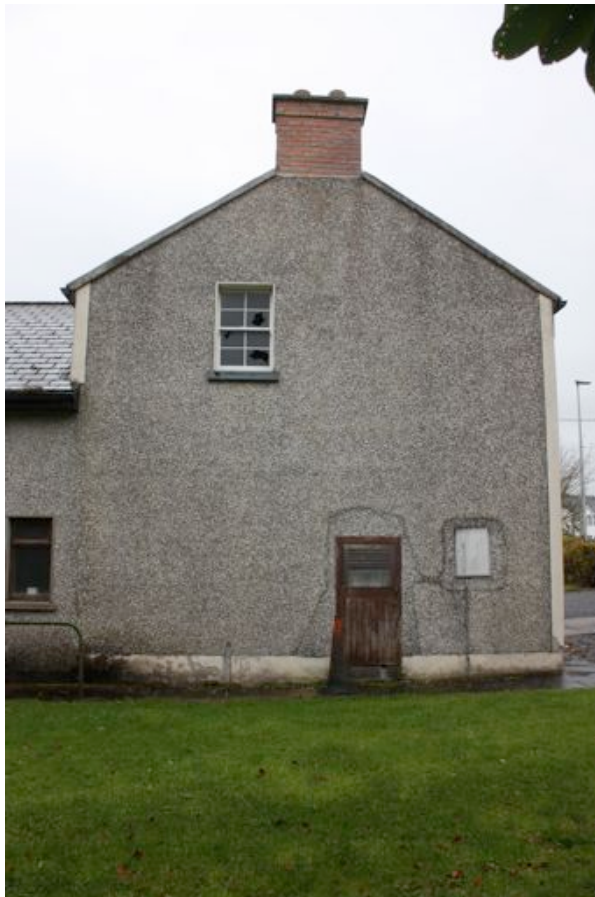
15. North gable of original house. First floor window with broken panes. The boiler room door and electrical meter may have been inserted after the house was pebble-dashed in 1987, hence the cracking in the render at these openings. There is severe cracking to the render at the mid span of the gable, the cracks visible through the entire wall thickness at first floor level.
