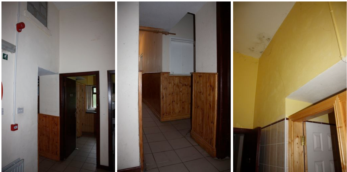
36. Lobby to toilet area. The rear wall to the original house is to the left, with the first floor stairs window infilled with blockwork at high level and the opening to the entrance hall below. 37. Opening into the original house, with entrance hall to left and hatch to kitchen in centre. 38. Toilets, the wall to the right is the rear wall of the original house, which was opened up to provide space within the original house for sanitary accommodation.
