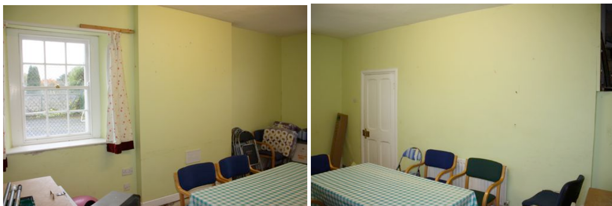
22. South wall with window and chimney breast, fireplace removed with vent in chimney. 23. North wall with original four panel door to left and hatch to stairs half landing to extreme right.
