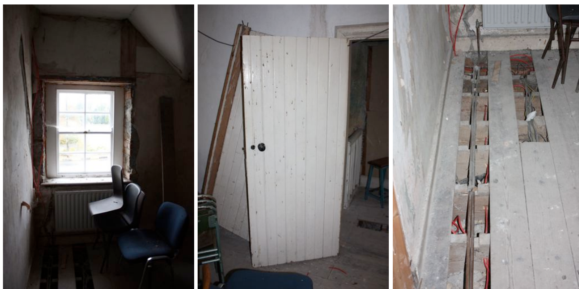
North-east room; 47. Window in north wall. 48. Original vertical sheeted timber door, with loose lying similar door behind. 49. Floor boards removed for plumbing and electrical installation.
