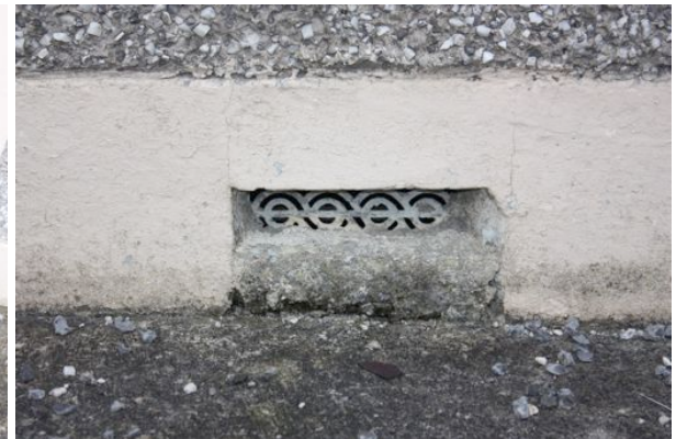
7. Entrance door threshold, with limestone slab. The outward replacement door continues below the door frames concealing the threshold. 8. Original decorative metal sub-floor vent.
