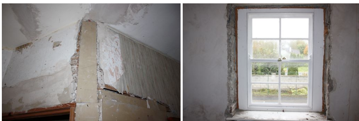
South room; 42. Original door to south-west room has been blocked with plasterboard, to right hand side. Original partition forming two rooms has been removed and the corner of the partition junction now chamfered in plasterboard. 43. Detail of west window.
