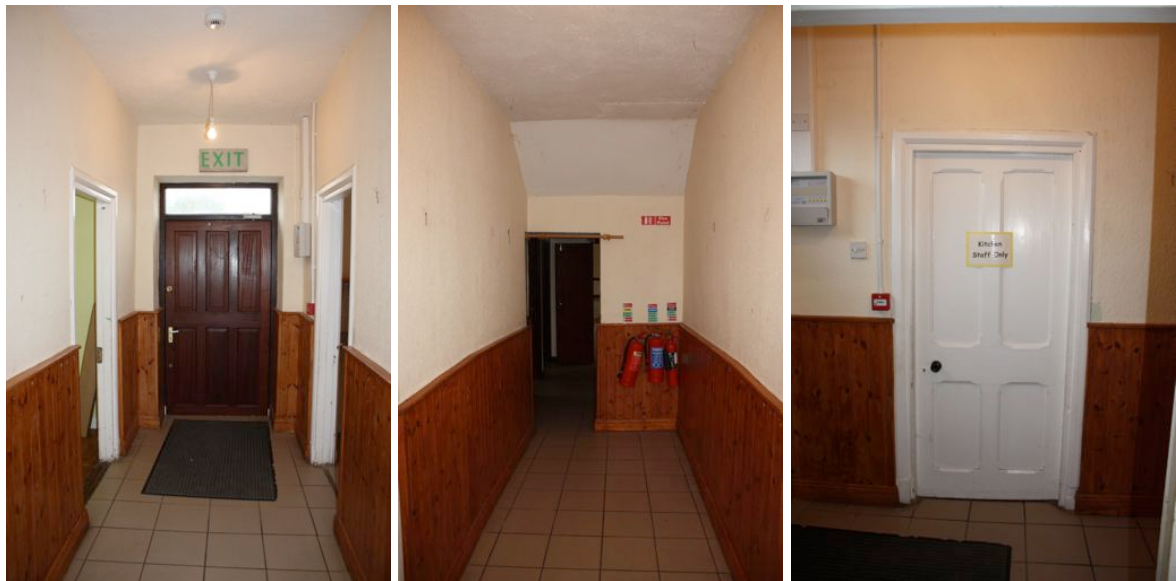
31. West wall with entrance door, door to north & south room to right & left. Modern timber panelling to dado level. 32. Opening to community hall, sloped ceiling to rear of room. 33. Original four panel door with chamfered detail to stiles and rails, moulded frame and chamfered architrave.
