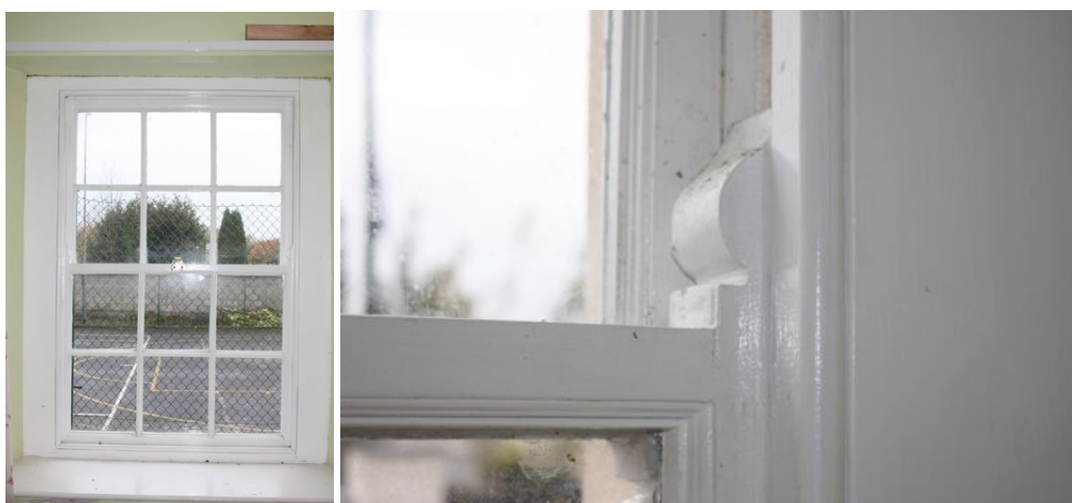
24. Detail of window in south wall. 25. Detail of carved window sash horn and moulded window frames.
