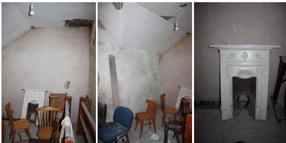
North-west room; 44. north wall has been drylined. Damage to ceiling. 45. North-west corner. 46. Original fire surround and mantelpiece, perhaps from south room.
