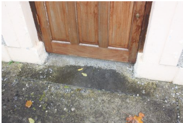
7. Entrance door threshold, with limestone slab. The outward replacement door continues below the door frames concealing the threshold. 8. Original decorative metal sub-floor vent.
