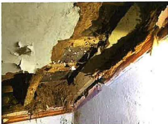
Part of the roof is supported by light timber posts. Complete new roof is required. Dry rot evident on roof timbers.
