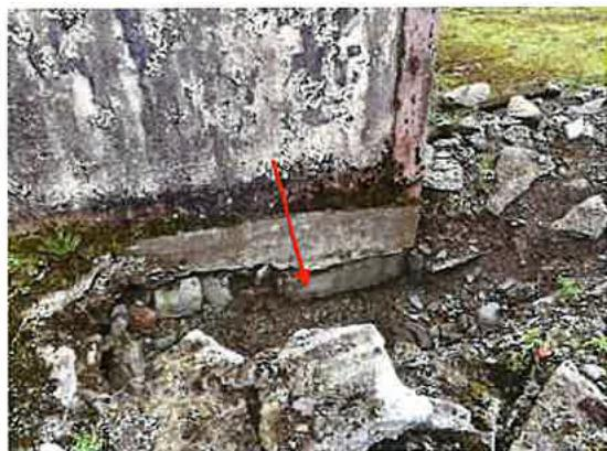
Also, noted that walls to the extension are merely laid directly onto the concrete yard and no foundation laid. Underpinning of the rear extension also required.
