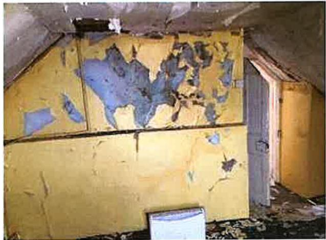
Moisture meter readings taken show high levels of dampness on all walls. All walls will have to receive 100mm external wrap insulation plus allowance will also have to be made for fitting Isover metal stud wall system on the internal face of all external walls and fitting 100mm insulation also.
