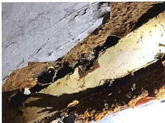
Also, noted that the chimney stack at centre of roof is in poor condition with substantial water ingress. Allowance will have to be made for demolition of the entire chimney stack from ground level and replacement with new.
