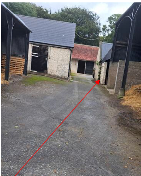
View of stable block in farmyard captured under inspection of 25/60577
