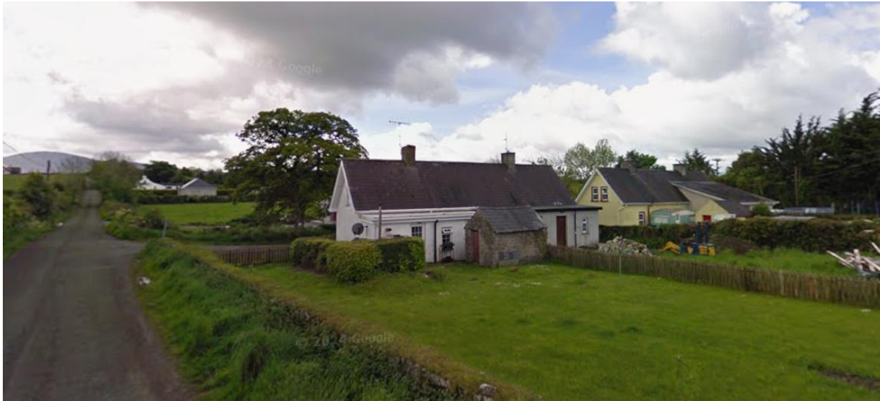
Figure 2 Rear elevation C. 2009 (Google Streetview)
