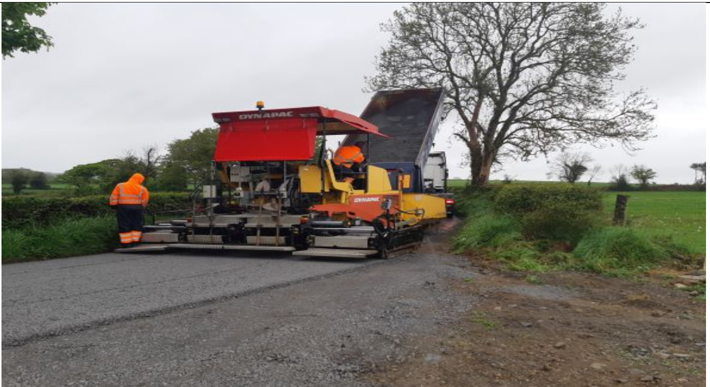
Resurfacing at Carrigagown South, Kilbarron, Nenagh – L-1099
