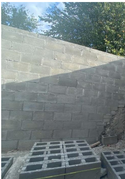
Figure 8 Interior structure under construction
